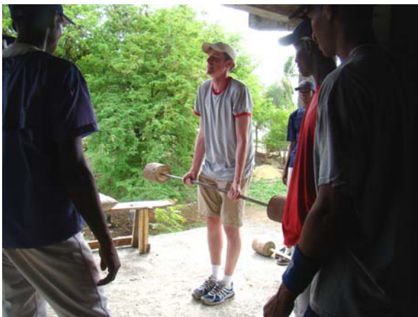
Sean Gregory pumping.....cement.
